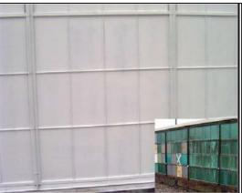
The Nano Ceramic Coating Systems product is used on the roof of metal frame workshop in Shanghai city, China. The roof temperature decreases 20°C in summer, and the value is 8.4°C in the floor of workshop (6m in height). The indoor temperature of glass house decrease 22°C in the summer.
