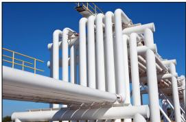
The Nano Ceramic Coating Systems product is used for the high temperature pipe to avoid burn (test), Hainan, China. The temperature of the pipe decrease from 89°C to 47°C with ~450um thickness product.
